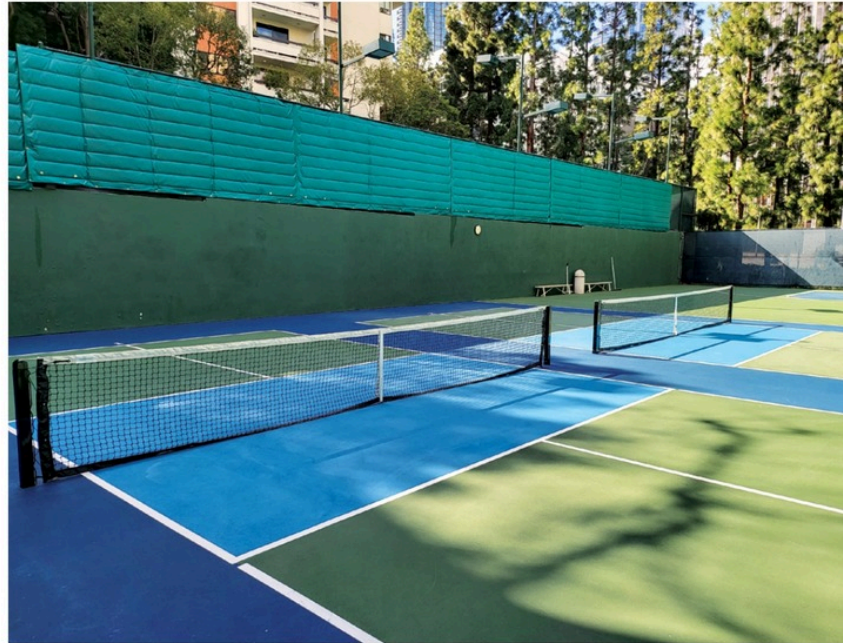
Environmental Noise Control installed its STC-25 acoustic blankets around this Southern California pickleball court to help ward off complaints about the noise that escapes from the courts. Image: Behrens and Associates Environmental Noise Control
