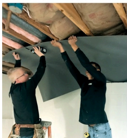
The classroom at upper top was originally designed to allow airflow for heat and air conditioning between classrooms, but this amplified the sound from room to room, creating distractions. The photo above shows the SoundSafe™ acoustical barriers from E Squared Technical Textiles being installed to mitigate this issue. Images: E Squared Technical Textiles
