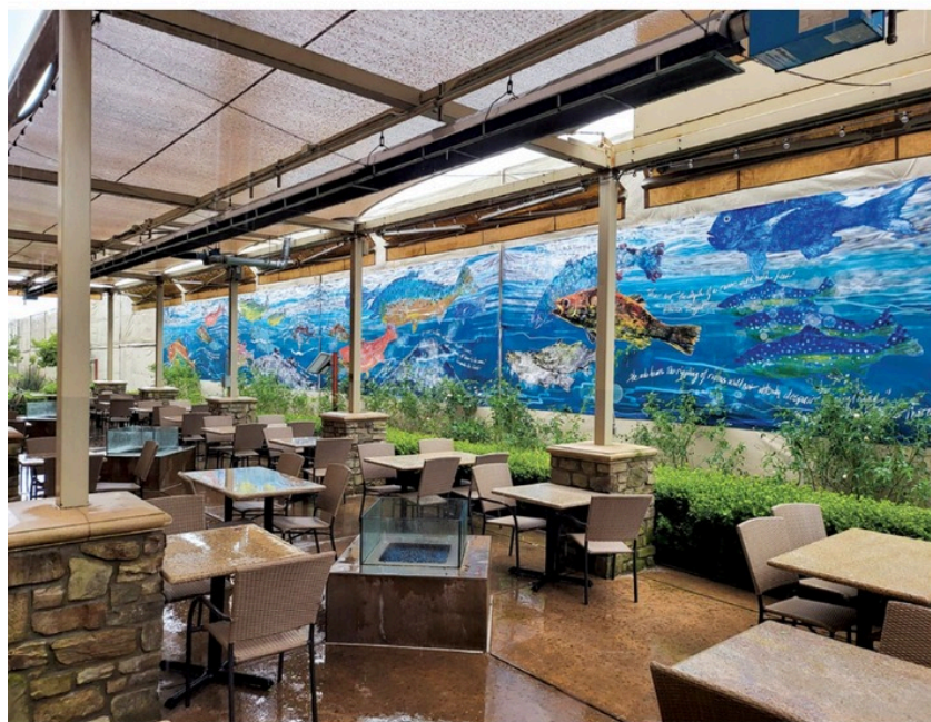
This acoustic wall from Environmental Noise Control was created by stacking together 8-by-20-foot panels to make a 16-foot-high wall with a graphic overlay. It was installed against the property line of a Hampton Inn in Sacramento, Calif., to protect hotel guests while a construction project was underway. Image: Behrens and Associates Environmental Noise Control
