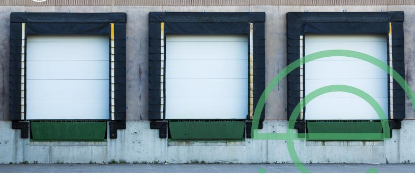
TPU's rugged durability and superior resistance to abrasion, punctures, and harsh environmental conditions make it the material of choice for dock seals. It holds up to repeated contact with trailers and extreme temperature swings, ensuring long-lasting performance in high-traffic loading zones.
