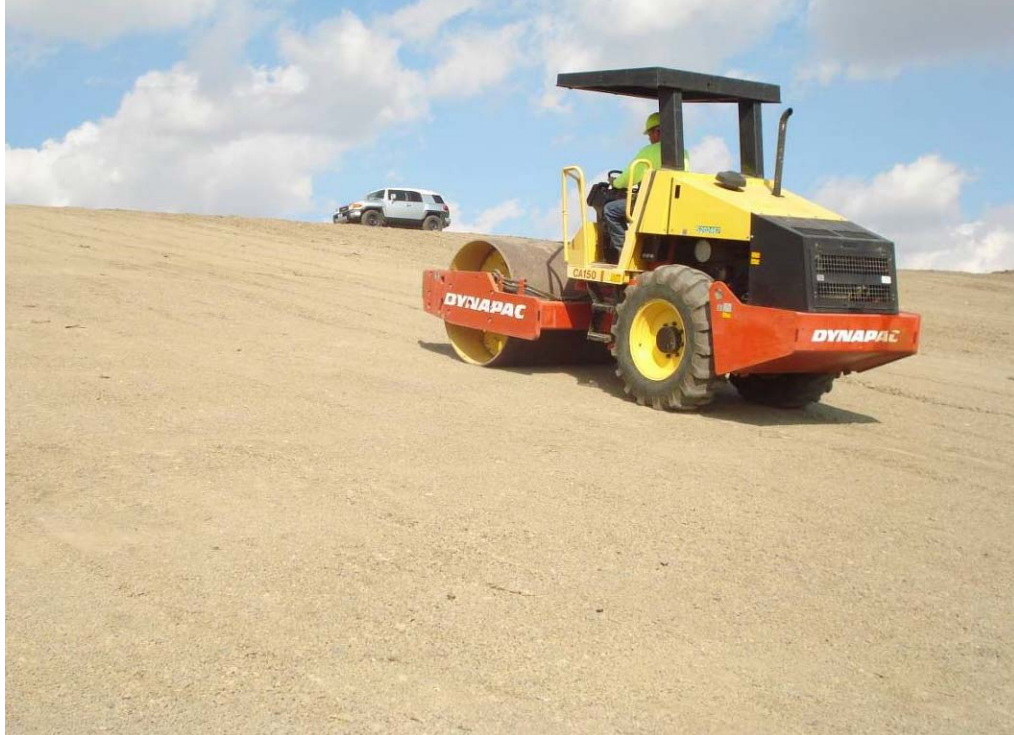
(a) Example of acceptable drum smooth rolled surface
