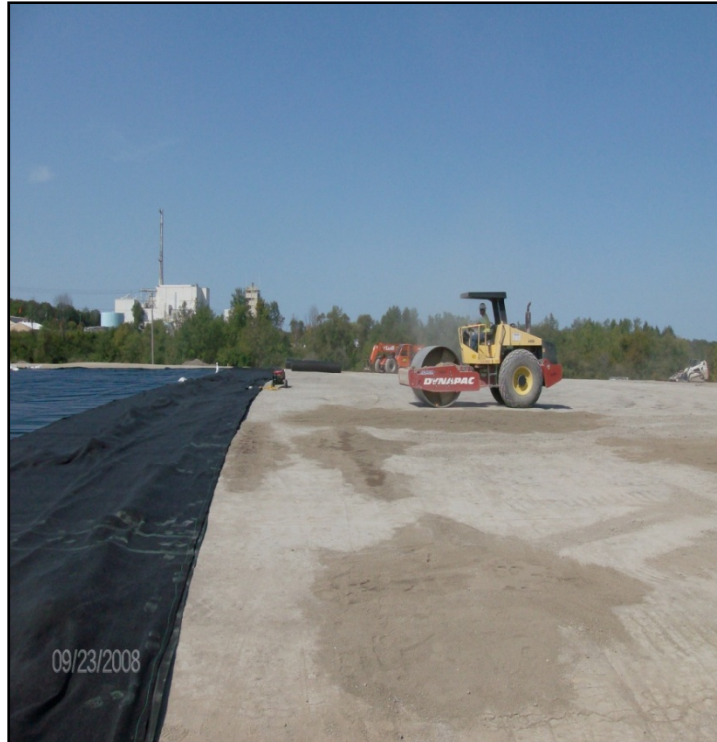
(c) Example of acceptable drum smooth rolled surface
