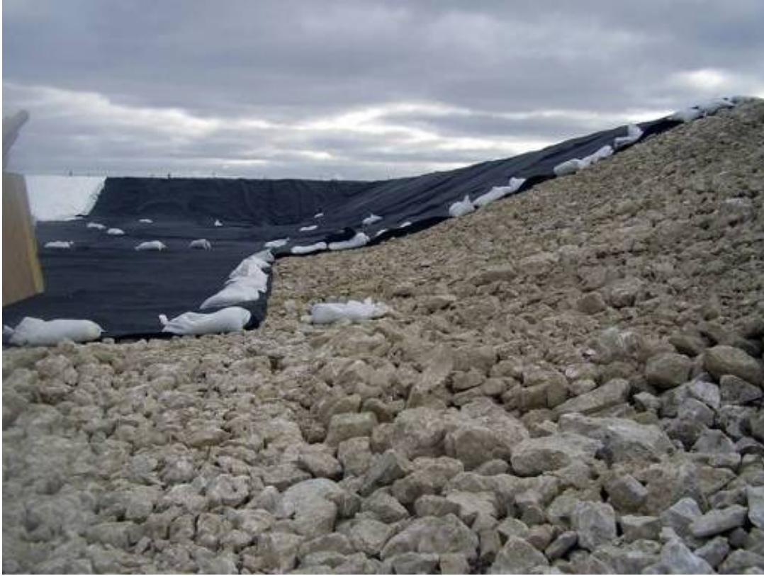
Figure 2: 0.75 mm thick PVC geomembrane with a geotextile protection fabric of 540 \text{ g/m}^2 being placed on a 100 mm-diameter ballasted rock subgrade.
