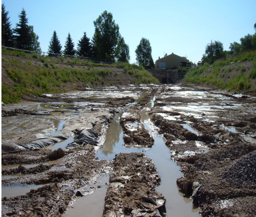
Figure 3: Unprotected subgrade damaged by flooding
