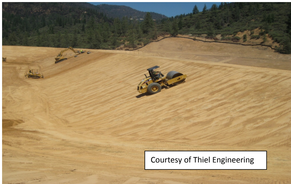
(b) Example of acceptable drum smooth rolled surface
