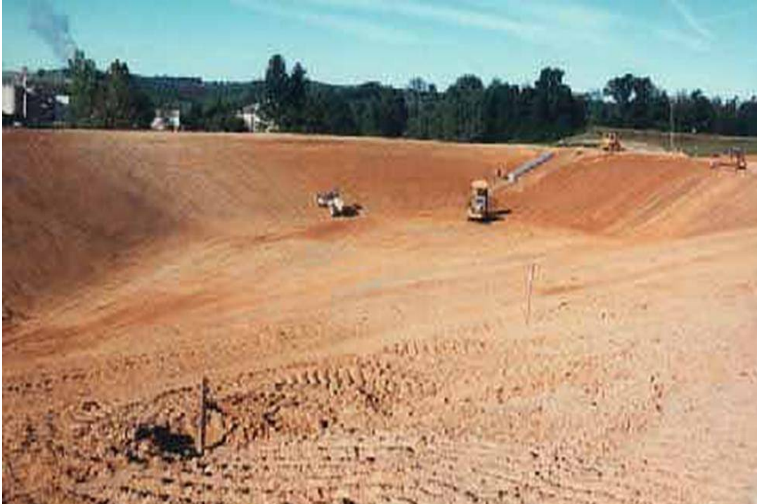
Figure 5: Almost-acceptable subgrade in the foreground.
