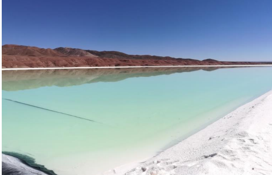
Figure 1. In-service evaporation pond for lithium mining (photo from Acevedo-Soriano and Cortes, 2021).
