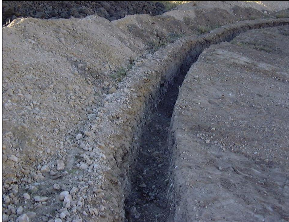
Figure 10. Excavated anchor trench in rocky material prior to geomembrane placement.
