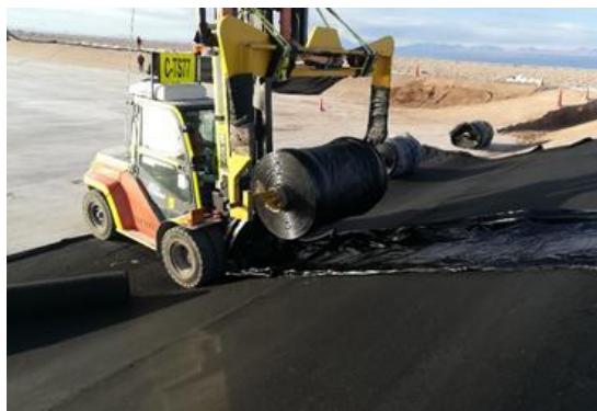
Figure 5. Suitable equipment for moving and unrolling a rolled geomembrane panel.
