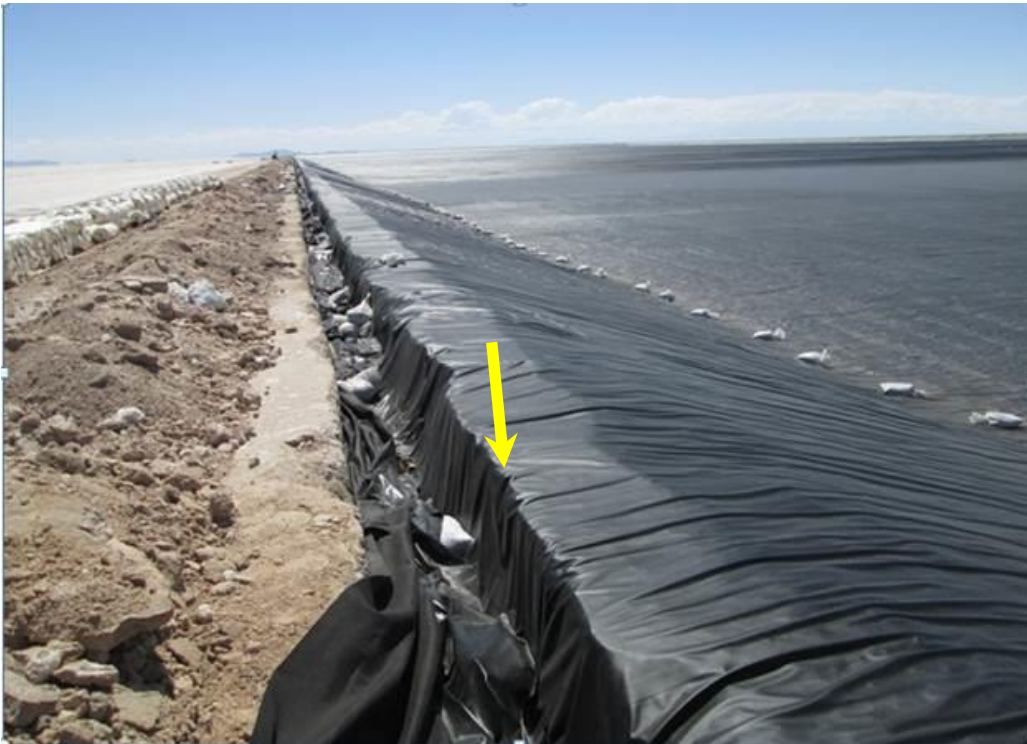
Figure 9. Upper edge of deployed panel inserted and ballasted in anchor trench.
